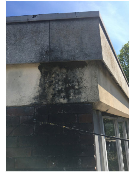
The main ring beam on the SW corner. The discoloured concrete indicates overflowing gutters and has led to spalling fabric and exposure of the steel reinforcement
