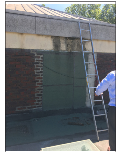
The ring beam shows signs of water damage and concrete spalling exposing the steel reinforcement
